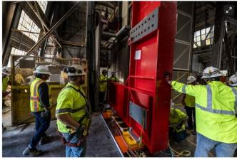
Supported from above by a crane, the L-beam is carefully moved into position by the rigging team for transport down the shaft in Lead, South Dakota. (Courtesy of Matthew Kapust, SURF)
