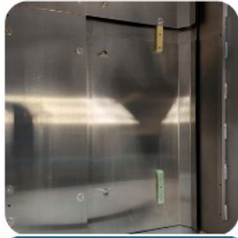
Vessel after installing two layers of shielding.
