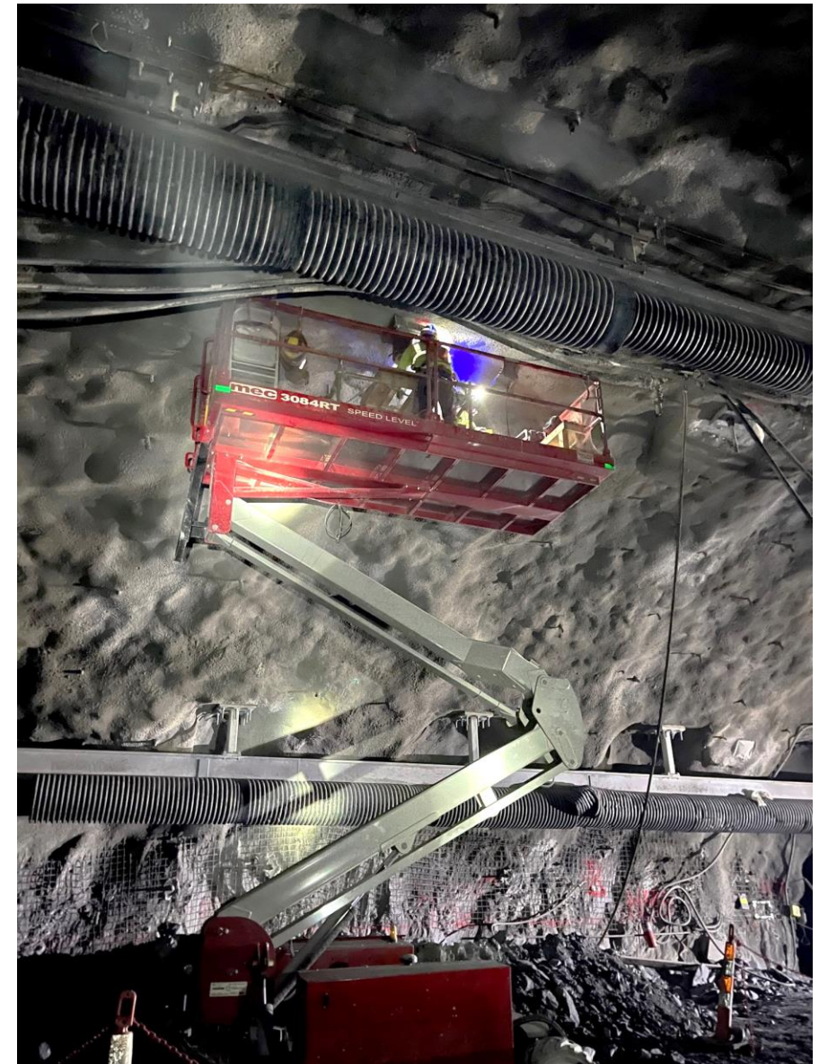
Extending monorails that will support material handling cranes in South Detector Cavern (4850-37)
