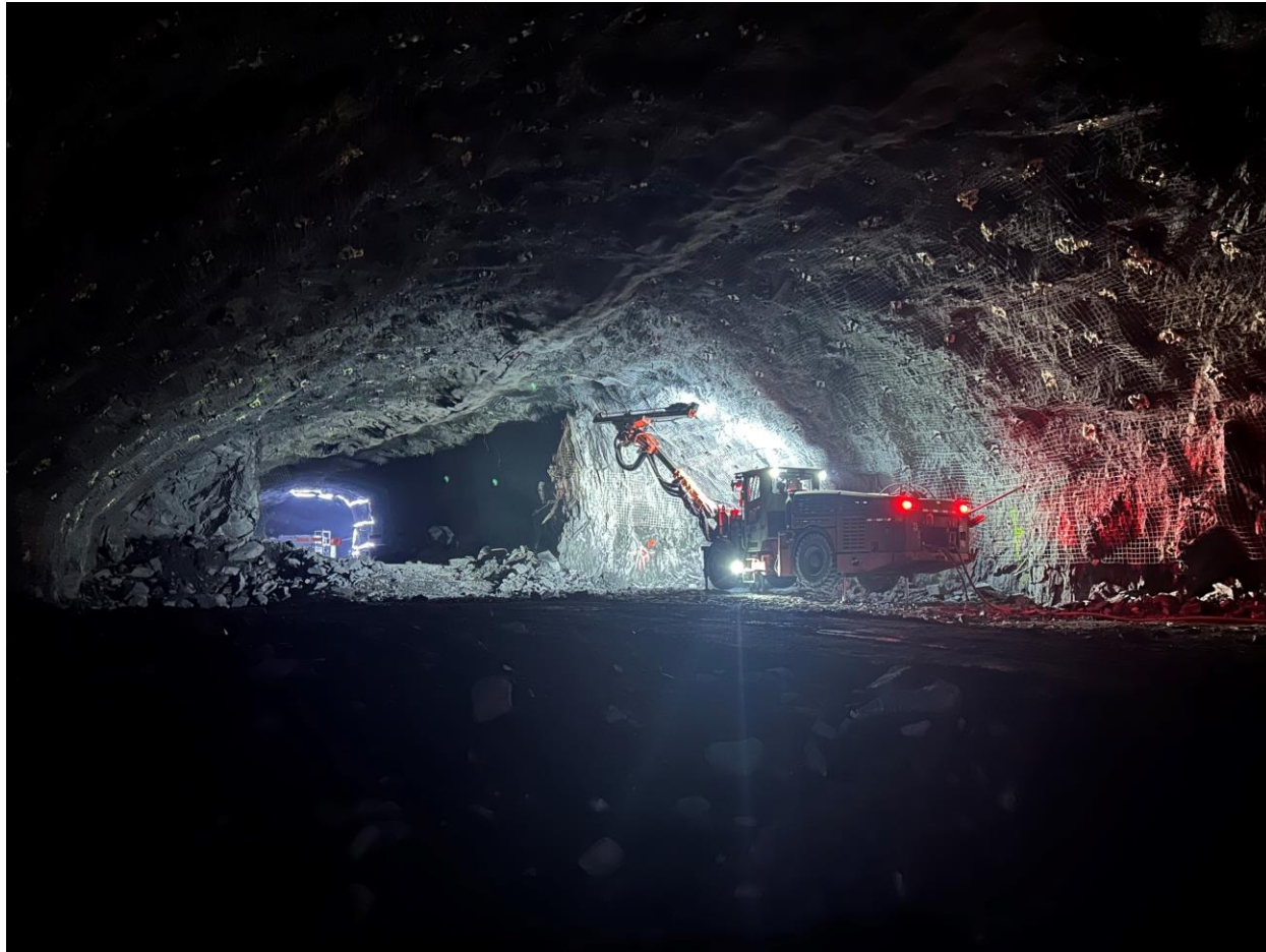
Drilling holes for blast charges in Central Utility Cavern (4850-36)
