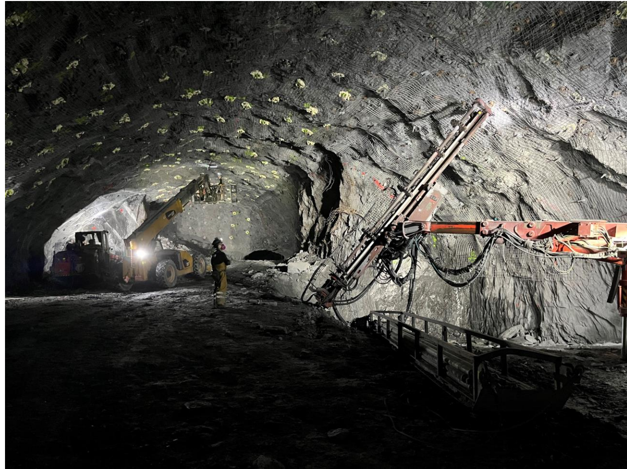
Installing CT Rock Bolts in Central Utility Cavern (4850-36)
