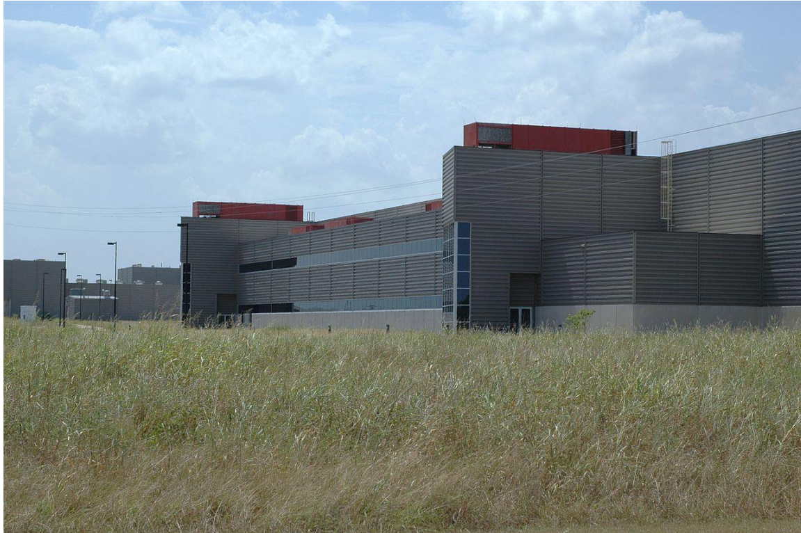
Magnet Development Laboratory building at the Superconducting Super Collider site in Waxahachie, TX, c. 2008. (Wikipedia)
