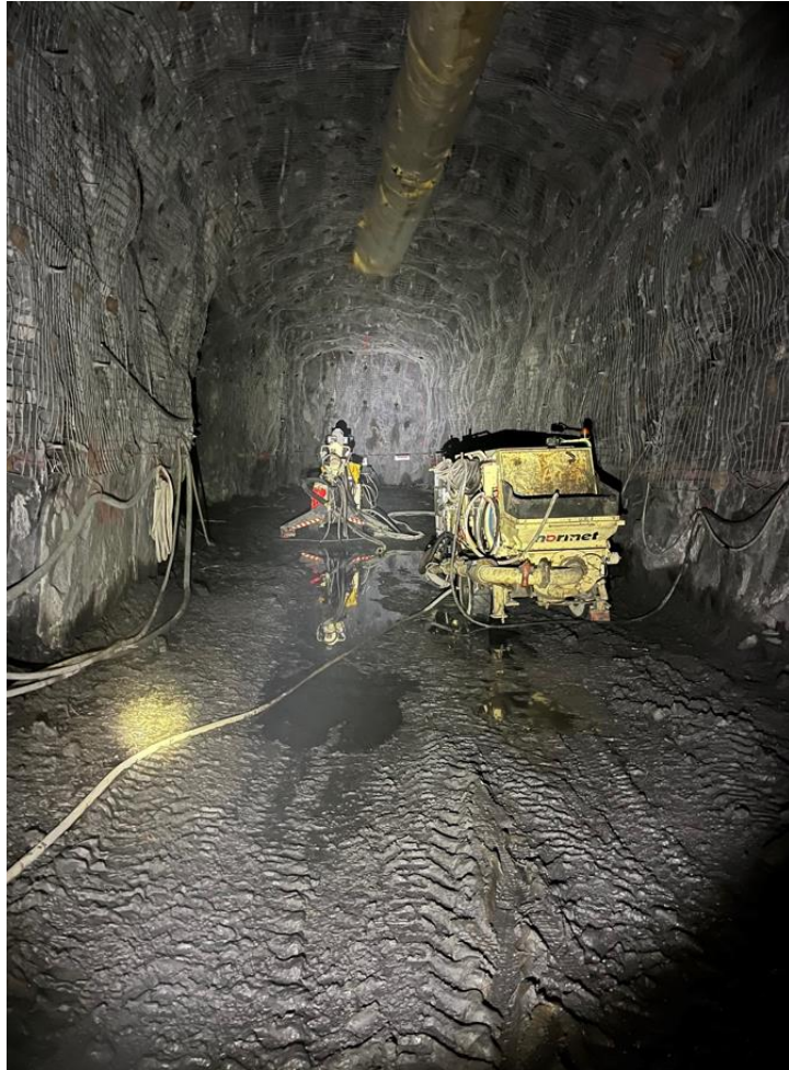
Setting Up the Robotic Shotcrete Machine
