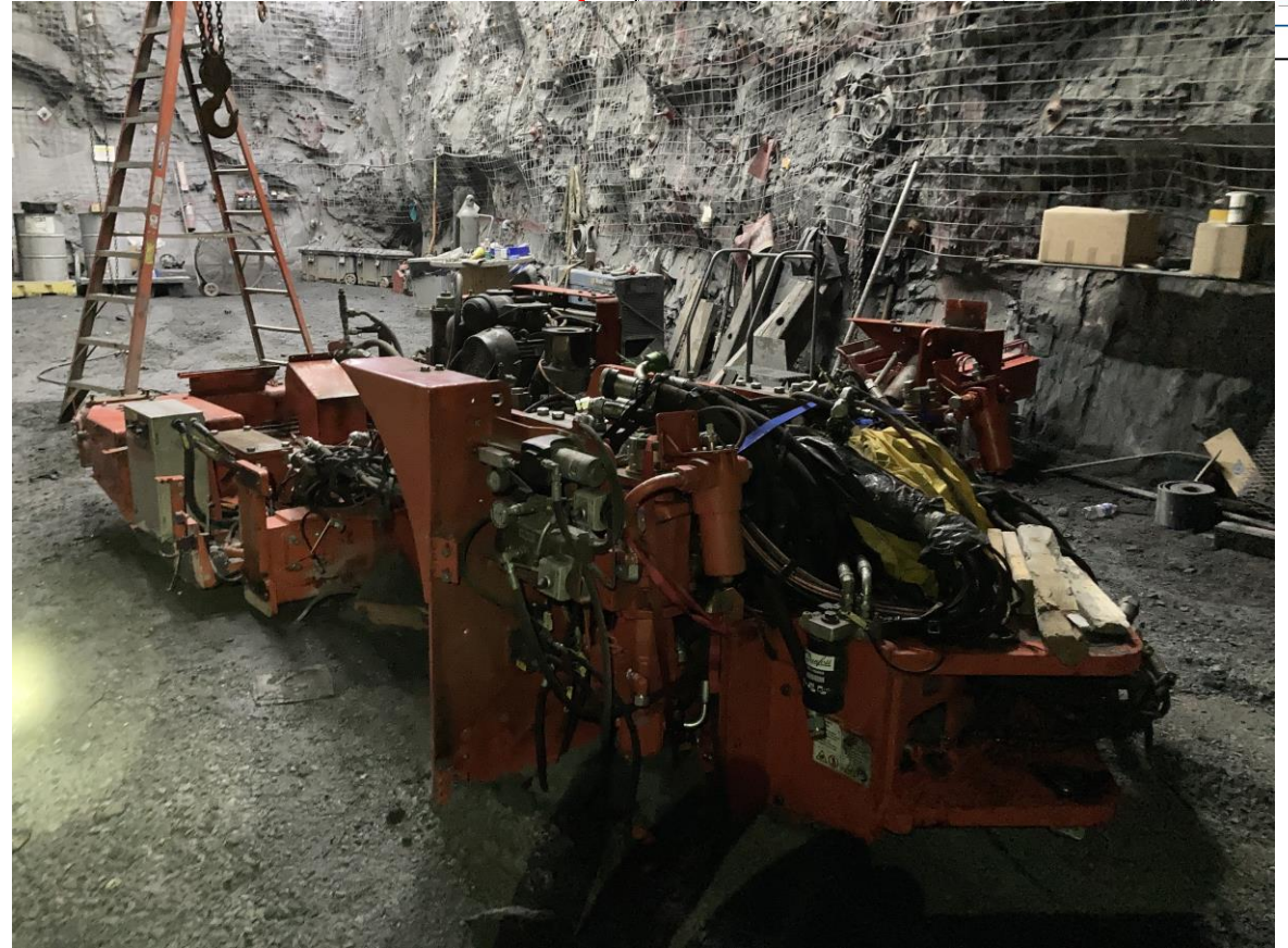
Sandvik 422i Jumbo being reassembled at 4850L in new maintenance cavern
