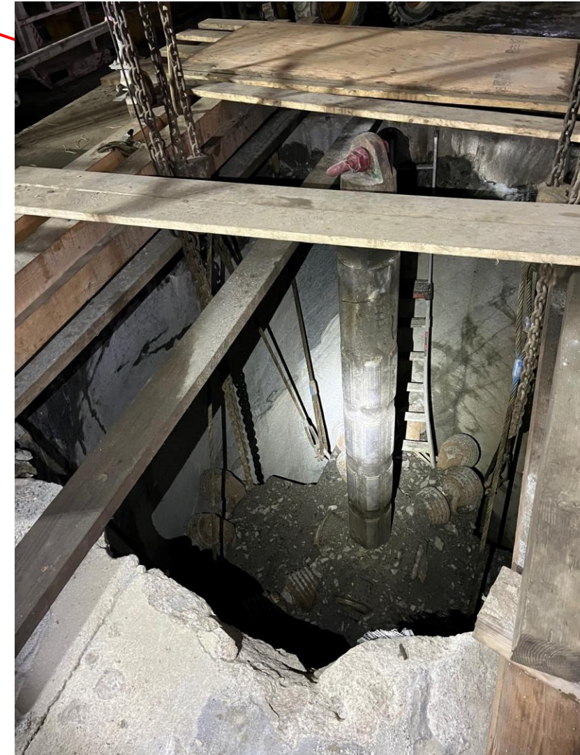
12' reamer head at breakthrough at 3650L Cavern – 4 Oct 2021
