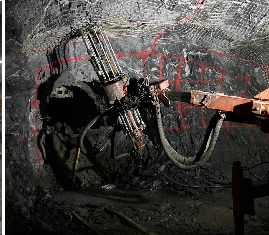
Installing rock bolts and welded-wire fabric for ground control
