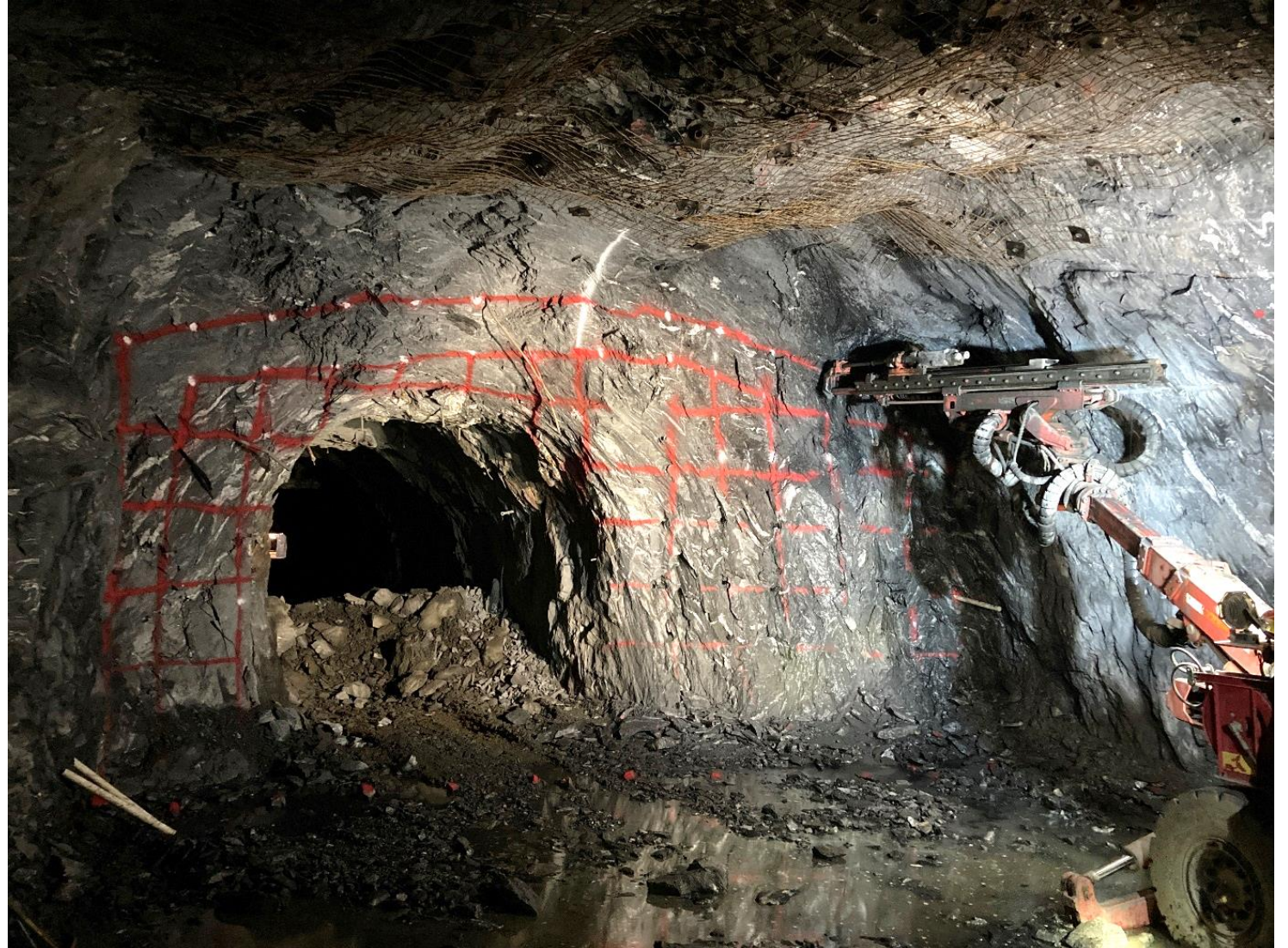
Drilling Charge Holes in the 4850-81 Face
