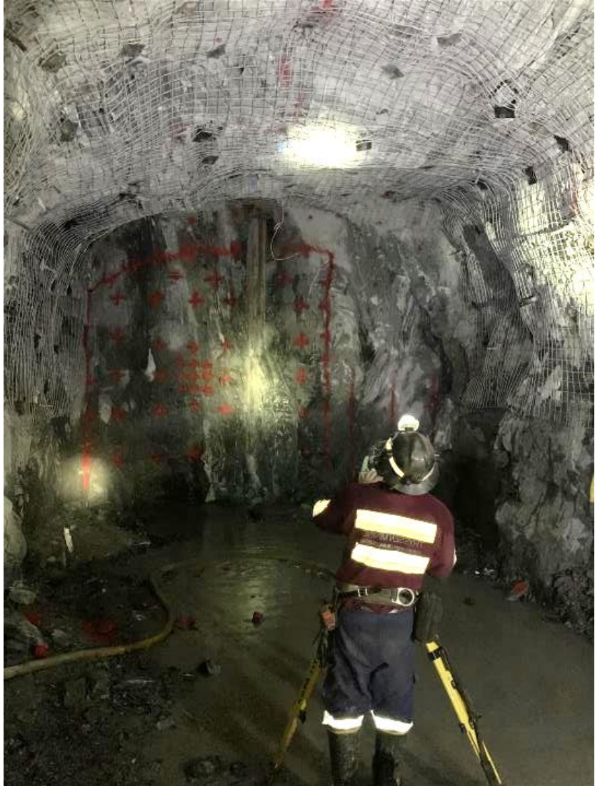
Setting out the Blasting Pattern
