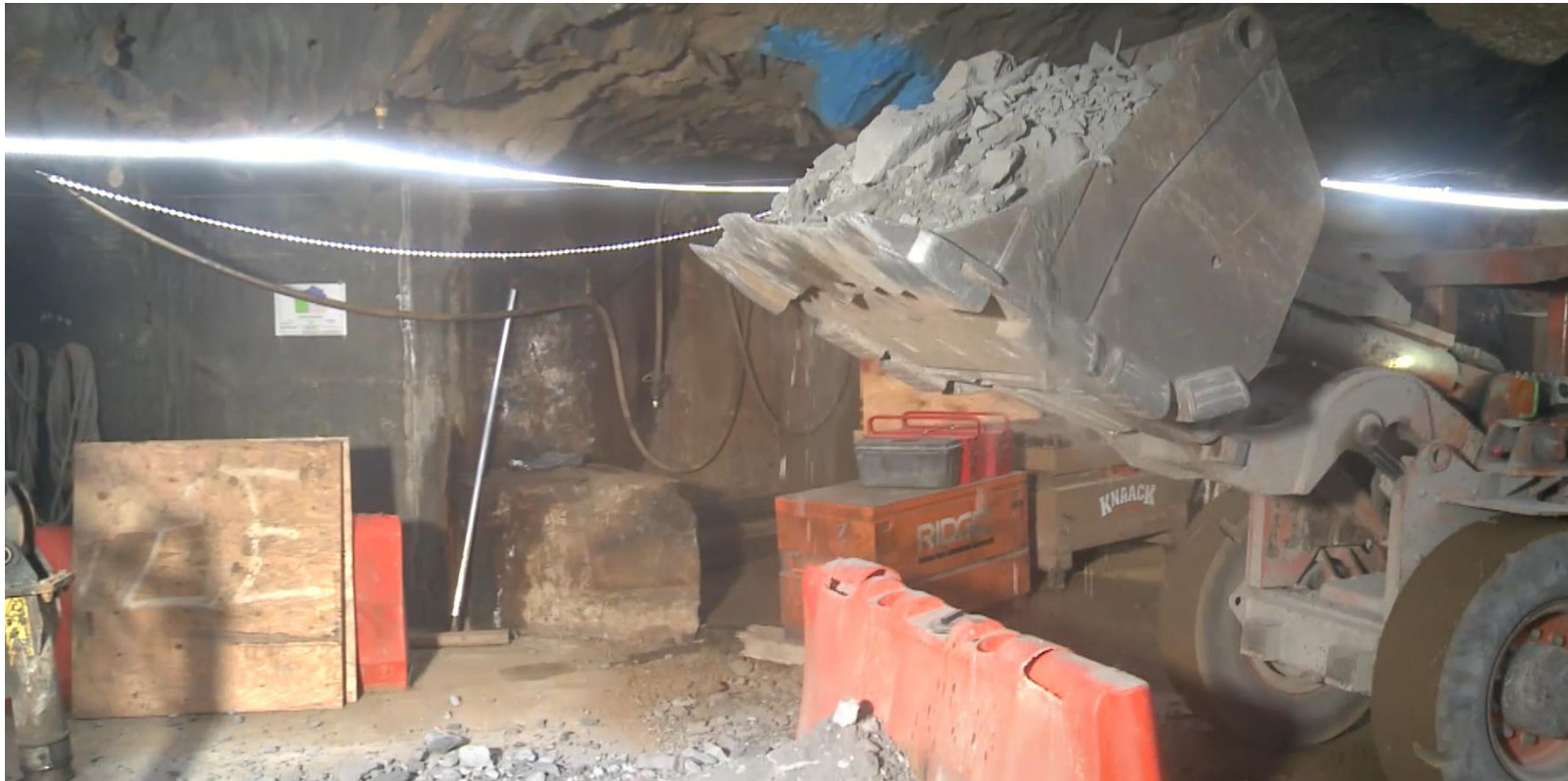
Moving “muck” to the ore bin, to be loaded in skip and moved to surface, crushed, and conveyed to the Open Cut
