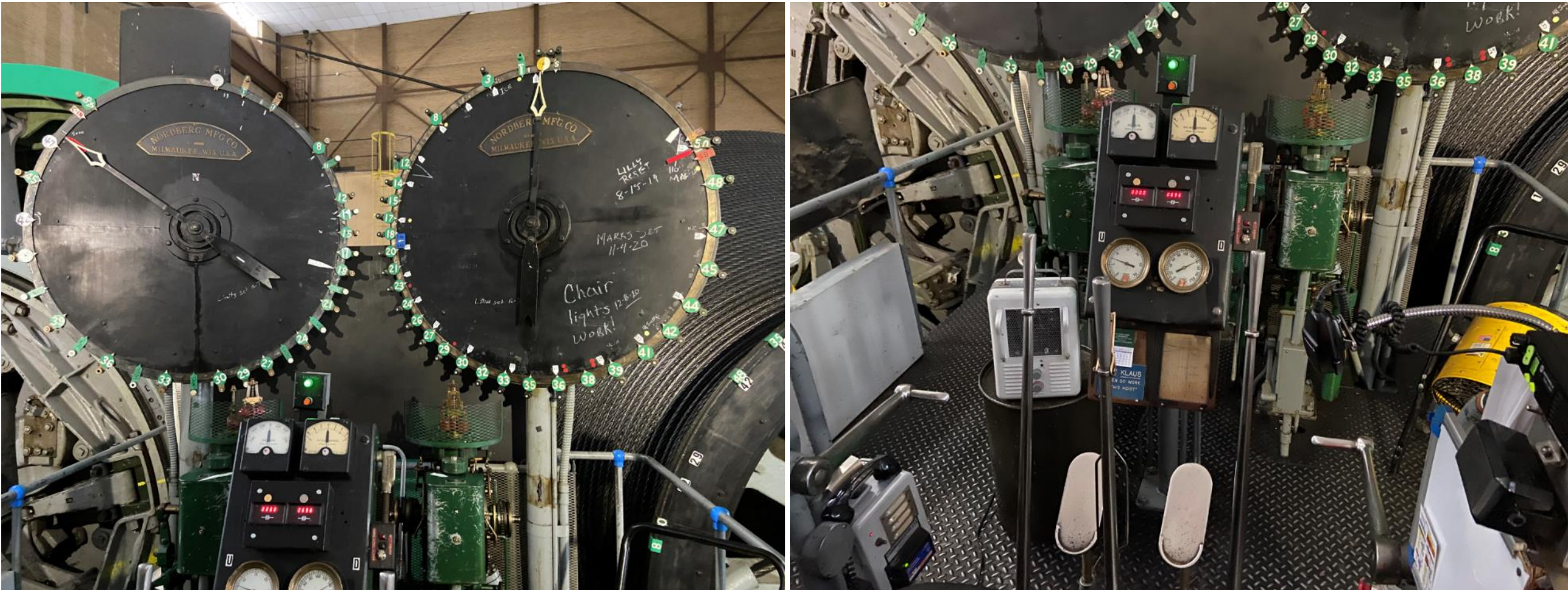
1930-era Control System - Foot Pedals, Analog Gauges, and Hand Levers - replaced with state-of-the-art digital control system
