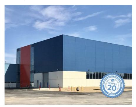
The new Industrial Center Building Addition received recognition as a new building that performs above code thanks to the design of its building envelope, which includes windows, exterior walls and roofs. The building envelope surpassed the award's criteria of a 20% improvement over current building code, providing a 25% improvement.
