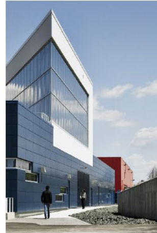
Illinois Accelerator Research Center February 2011
