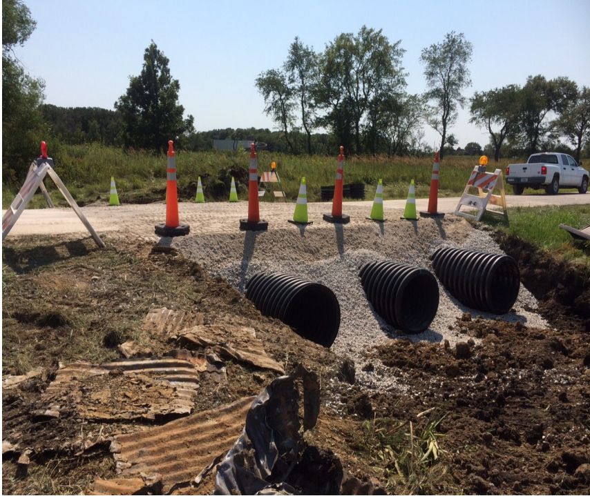
Culvert replacements under Batavia Road
